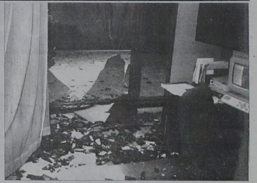
SHREDDED GLASS litters the desk and floor of Mike Schueler's office in Oklahoma City. He was not in the office when the bomb exploded. See story for details.
