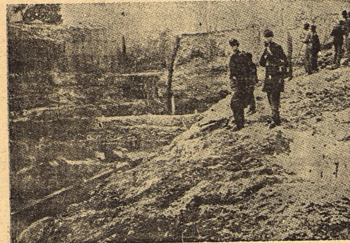
TO AVOID CONFEDERATE batteries at a bend in the James River, the engineers dug Dutch Gap Canal near Richmond, Va. This constituted a major task in view of the lack of mechanical earth-moving equipment during the Civil War.
