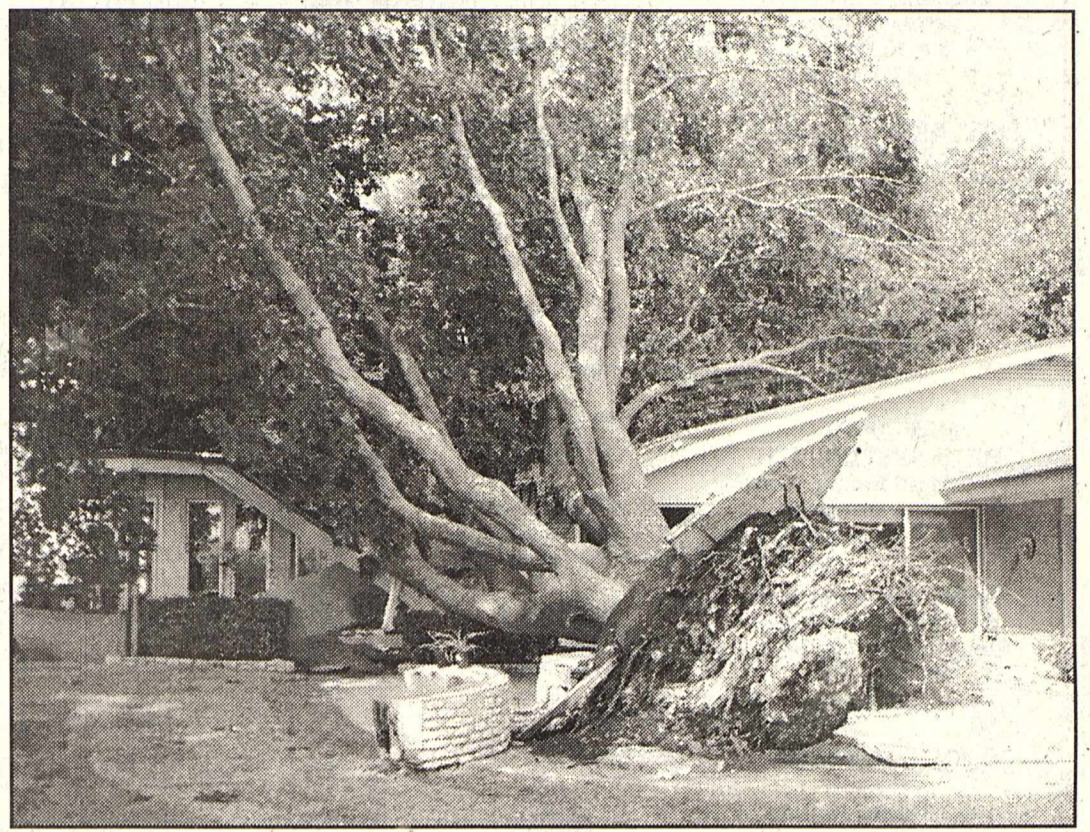
Howorth home damaged by uprooted tree.
