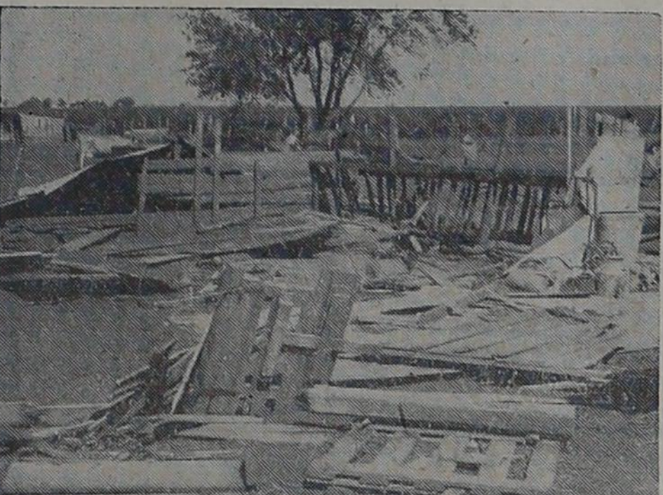
This is all that remained of the cow barn on the E. H. Meeks farm, in Oklahoma Lane community, when the twister struck there. It was a 15x40 frame structure and was located a few hundred feet south of the Meeks home.
