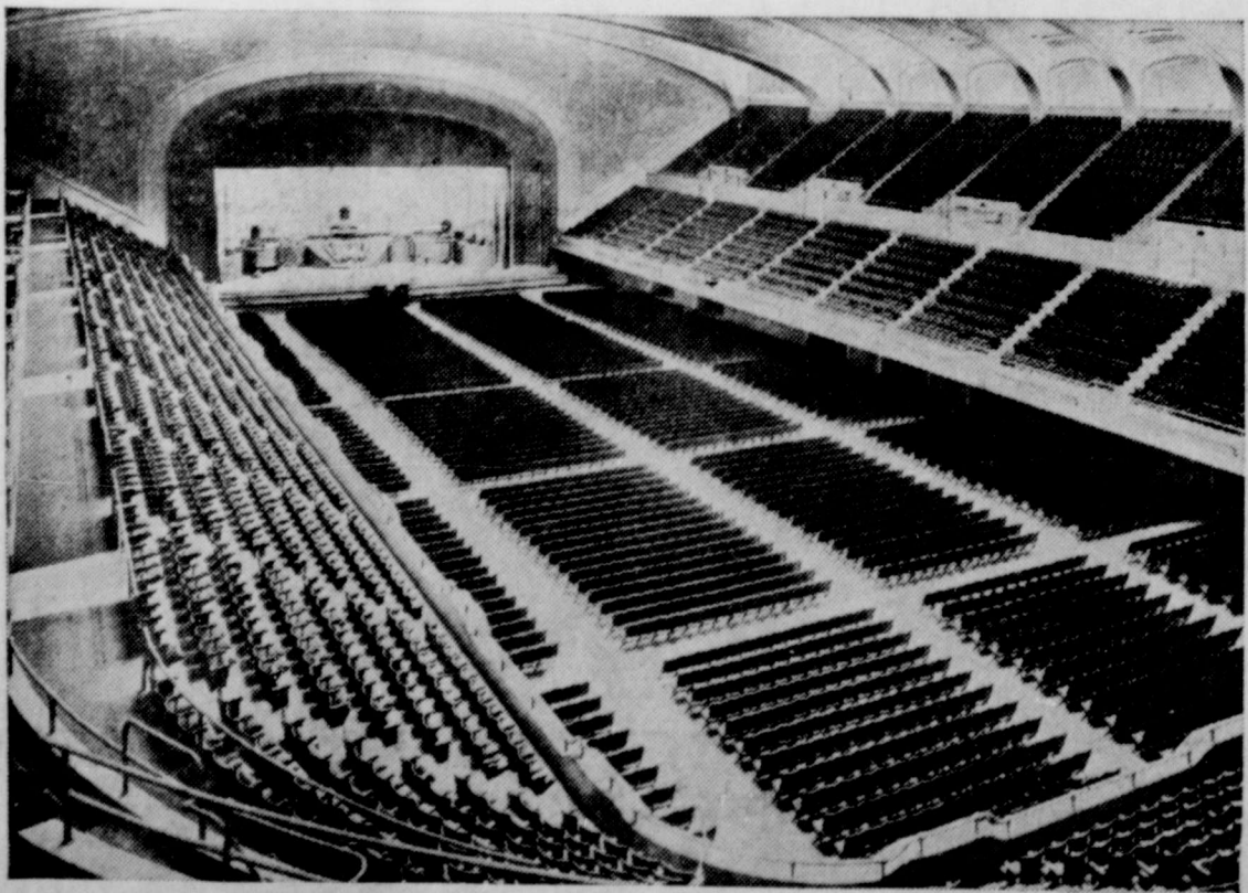
Interior view of the $7,000,000 Public Auditorium in Cleveland, Ohio, which will house the Republican national convention next June. The hall has a seating capacity of 9,000.
