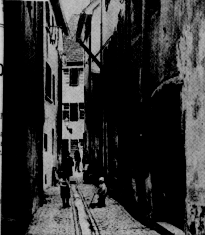
Clear Water Runs Through This Freiburg Street.
