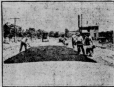
From Good Roads Magazine, New York. LAYING OUT THE ASPHALT.
