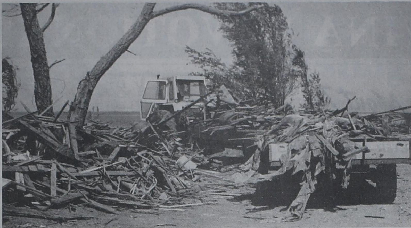
STORM'S RAVAGE... The debris left by the twister that hit the Marvin Mimms place near Lazbuddie resembled bombing damage. Trailers were employed to pick up the debris.
