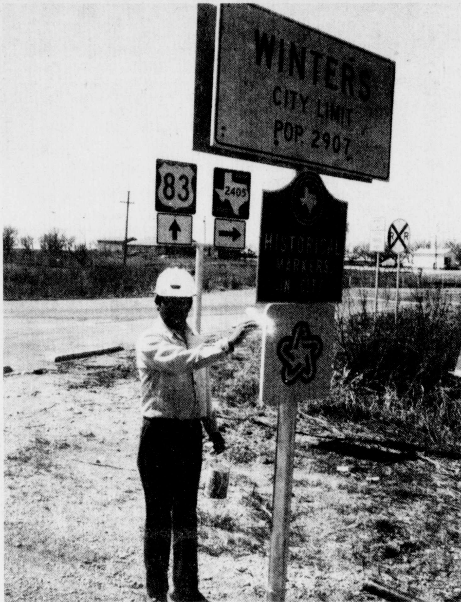
BICENTENNIAL—Julio Galvan Jr., maintenance technician with the Highway Department, puts finishing touches of paint of the highway sign
