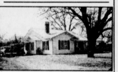
607 Bowen—3B/1B, dining, remodeled kitchen, central heat, fireplace, siding, carport, storage bldg., privacy fence.
