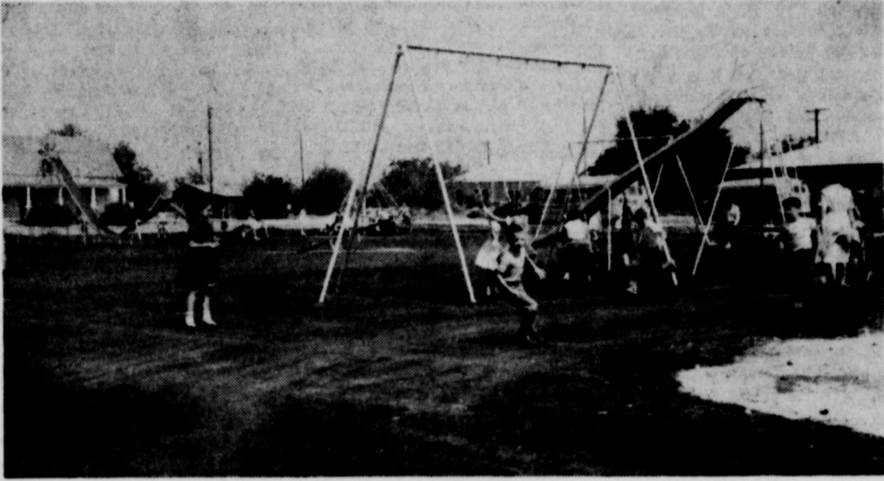
SCHOOL IMPROVEMENT — The playground used by the lower grades in Bronte Elementary School has been given a black-top treatment, eliminating much of the dust and loose gravel which have covered it in the past. At the lower right hand corner of the picture, is a small spot which was not treated. It shows the contrast of the old and new surfaces.
