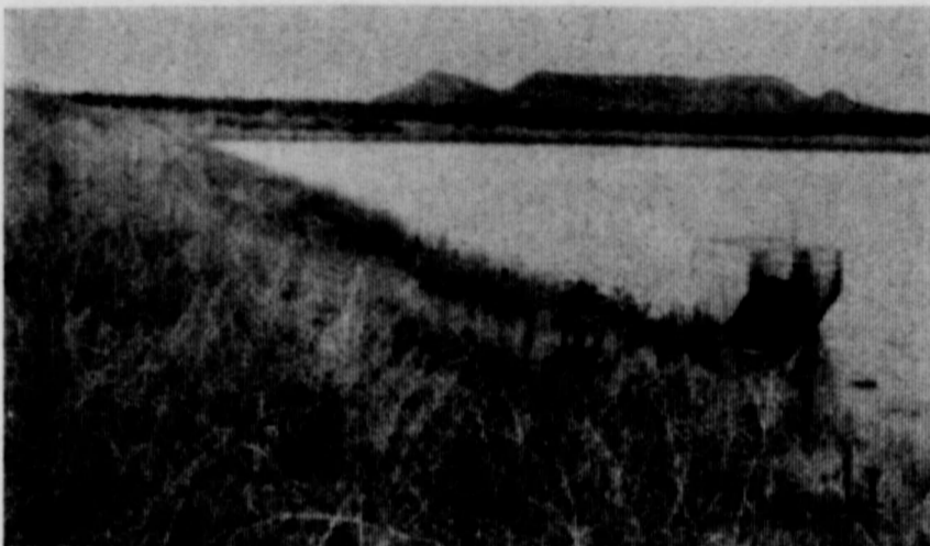
BEAUTY IN WEST TEXAS — A lake of water anywhere in West Texas is a thing of beauty, particularly when it does double duty to prevent flooding in the area below. Here is Structure No. 5 of the KWCID project. Note the luxuriant growth of grass at the left on the dam. The structure in the edge of the water is the spillway which allows flood water to draw down gradually and remain within the existing creek channel, thus preventing flooding below.
