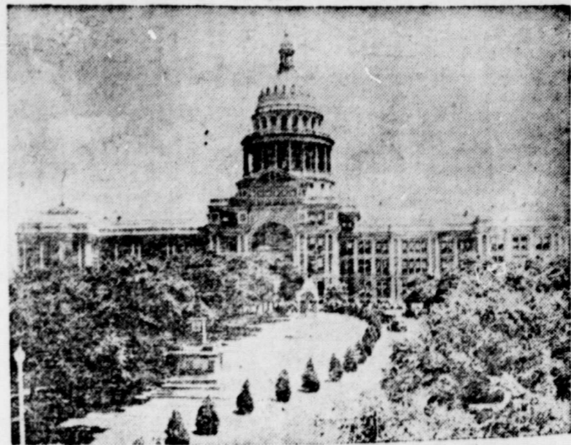
Largest and finest of all State capitols is that of the State of Texas in Austin. Constructed of Texas granite, its dome reaching seven feet higher than the national capitol in Washington, the Lone Star capitol is being visited daily by Centennial visitors from all sections of the country. Texas paid for its magnificent building a half century ago with three million acres of its far-flung domain.
