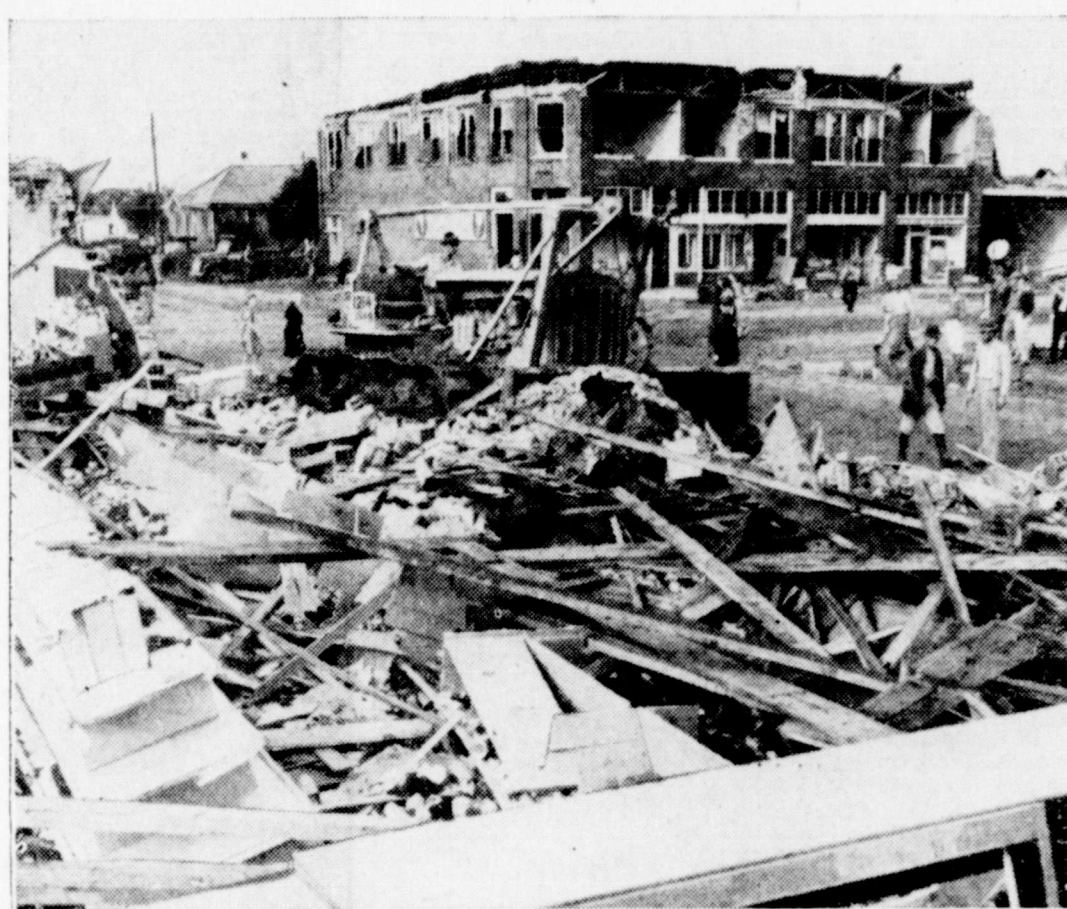
TORNADO'S HAVOC—With more than a third of its buildings hit, and a property loss estimated at over $2,000,000, town of Pryor, Okla., still removes wreckage wrought by tornado. The mass of broken wood and rubble in the foreground was once town's largest grocery store.
