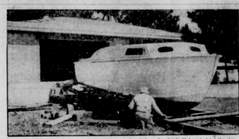
NO BOO-BOO, THIS—it was done on purpose. A switch on the classic "I forgot about the size of the door" theme, this 26-foot craft was built inside the nearly completed house with intent. Wiling hands help start the creation of Bob Brown, of St. Petersburg, Fla., on her way to water. Brown thoughtfully left installation of his picture window wait until "launching" of his ship.
