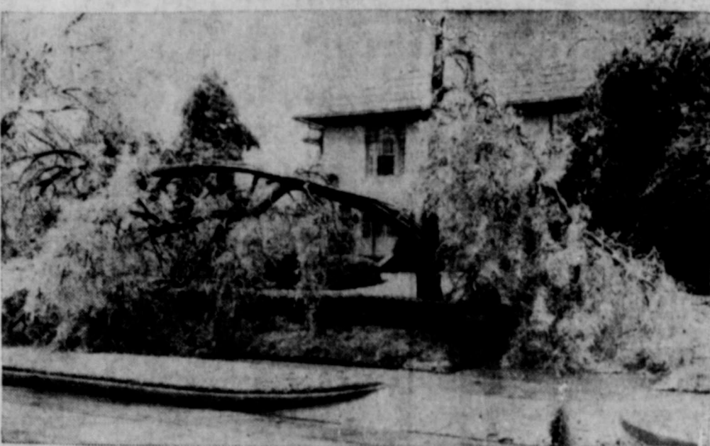
ICE STORM DAMAGE
