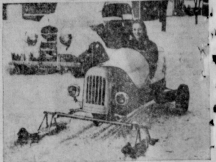
Ideal for driving during heavy snowfalls, this midget car, built in Athens, O., has a set of front axle skis, which can replace the front wheels. Called the "King Midget," the car was first put in production in 1946.
