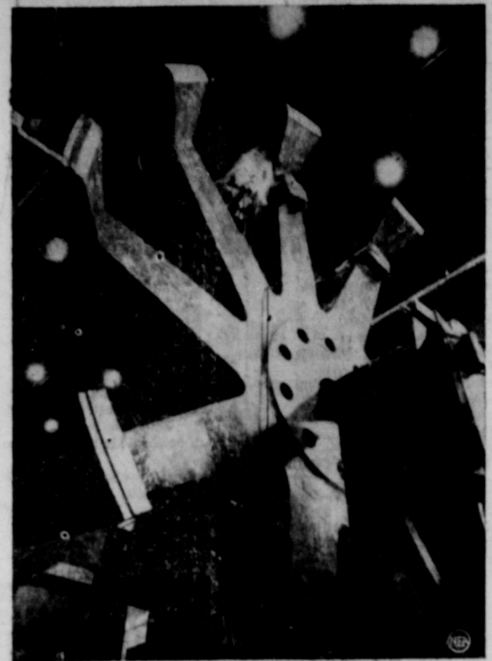
GIANT "SPIDER" —Little Miss Muffet would have been aghast if this 79-ton "spider" under construction in Pittsburgh, Pa., had sat down beside her. The "spider" is the inner framework for a 108,000-kilowatt waterwheel generator being built by Westinghouse for the Grand Coulee Dam power plant. A welder at work atop one of the "legs" is barely visible. When completed, the rotor will be 31 feet in diameter, will weigh 542 tons and will spin at the rate of 120 revolutions per minute.
