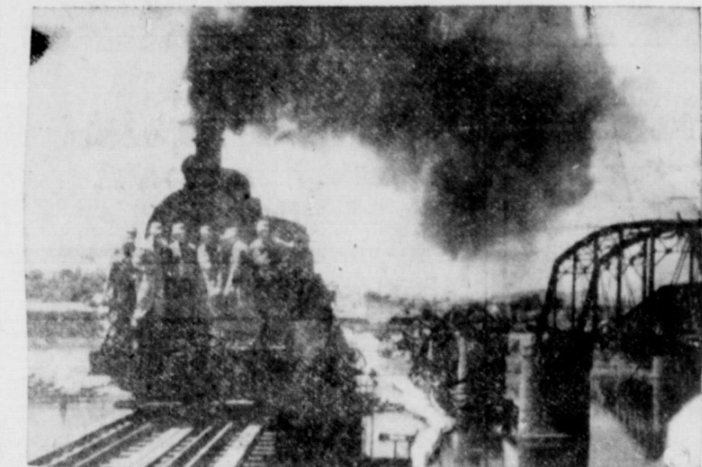
SERVICES RESTORED—Lt. Gen. James A. Van Fleet and Lt. Col. Barber, U. S. 8th Army are among those riding on the first train to cross the Han River on the newly reconstructed Han River railroad bridge. At right is wrecked Han River bridge. (NEA Telephoto).
