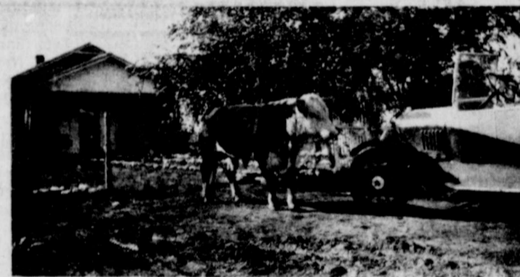
THE BROWN HOME PLACE — Portions of this adobe house, built by Frank Brown's grandfather in 1925, are still standing six miles east and three miles north of Lockney. The Brown family lived in the house until 1949. The house had three bedrooms, a living room, dining room, and back porch. The walls were 14 inches thick.
