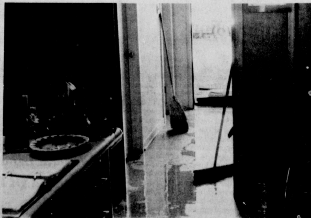
RAINS ON SUNDAY night left Miller Insurance office filled with water.
