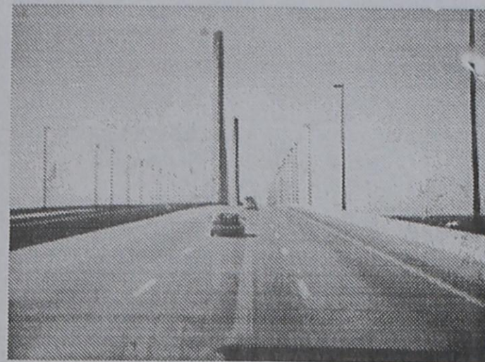
New bridge going over Chesapeake River in Delaware. The river flows into the Atlantic Ocean.
