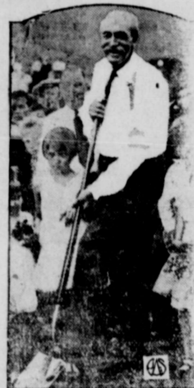
Governor Pinchot dug the first spadeful when work was begun on the Pymatuning dam, 25 miles above Sharon, Pa.
