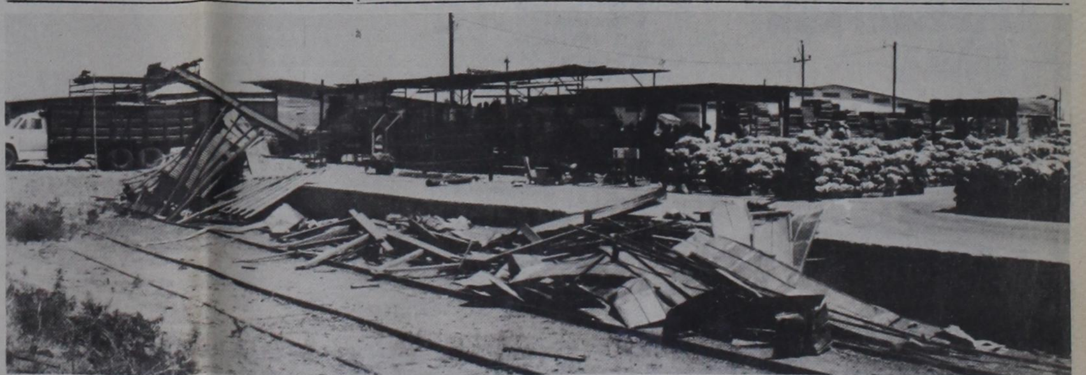
BACK IN BUSINESS—With tornado rubble pushed aside, workers for La Mantia, Cullum, Collier & Co., Inc., process onions where the east end of the big warehouse building used to be. Weather covers were built over the company's big onion processing machine—which was left relatively
