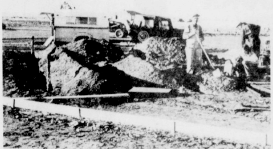
WORK PROCEEDS... Footings have been dug in preparation for pouring the foundation for the Friona Nursing Home, which is getting underway in the northern part of town.
