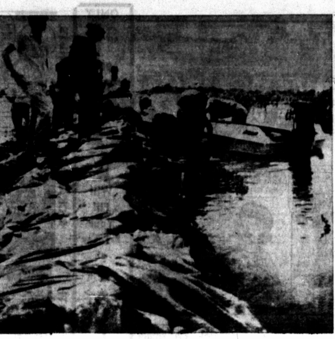
Volunteers used sand bags brought by boat to reinforce a weak spot in the levee at Port Acres, Tex. Many of the community's homes were flooded by two levee breaks which have been repaired by the volunteer sand bagging. (AP Wire-Photo).
