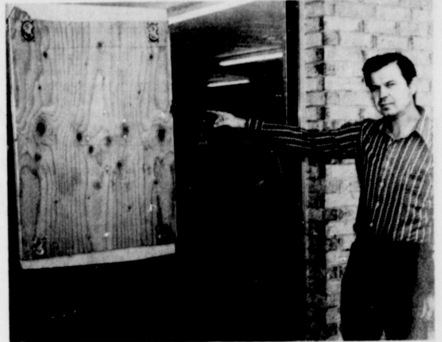
BROKEN WINDOW.... Leland Hutson, owner of Friona White's Auto Store, points to the display window which was broken out at his store for the second time this year. Merchants have set up a $500 reward for information leading to conviction of those responsible.
