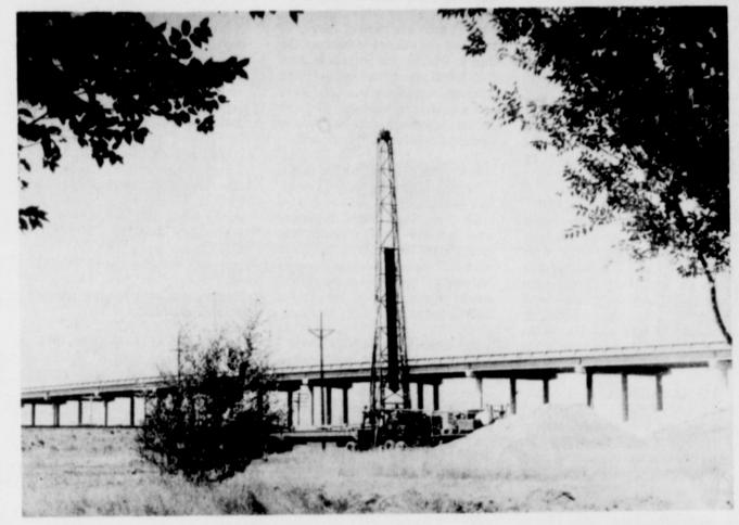
DRILL WORK STARTS....Drilling began on the new city water well at the southwestern corner of the city this week. The drill rig can be seen, with the overpass in the background. Big T Pump Company is the driller. The well is expected to be about 330 feet deep, and is located at what would be the corner of First and Ashland Streets. (Photo by Stanley Ellis)
