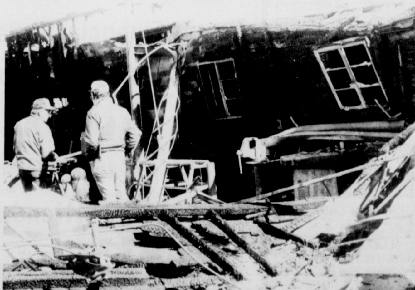
FIRE AFTERMATH....Waymon Wilkins, left, and Gary Renner are shown in the rubble that remained Monday morning following a pre-dawn fire which razed the shop area at Adams Drilling Company. The company's offices also were ruined. Plans are being made to rebuild.
