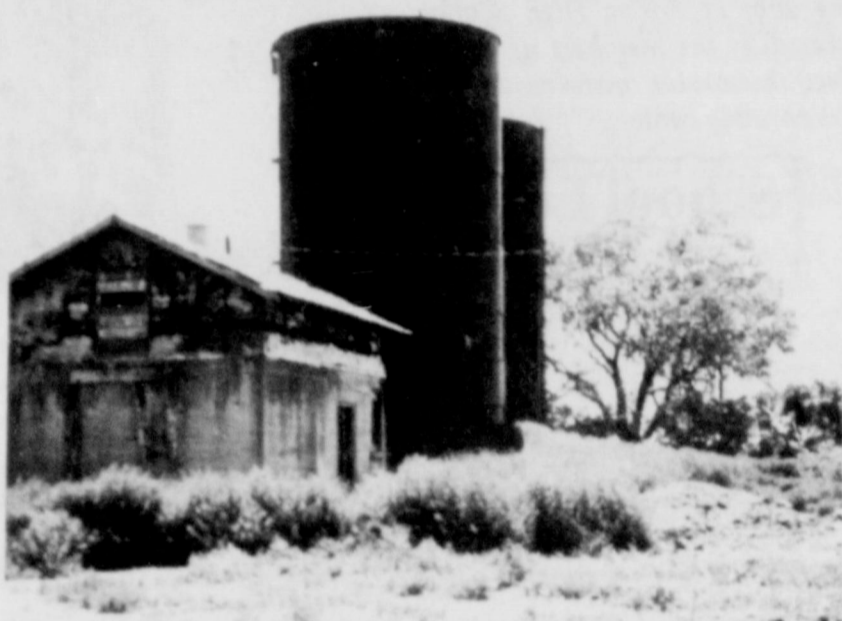
HOBO DEPOT.... In the late 1800's and early 1900's water tanks such as these, which are just west of Black, were often times called the "Hobo Depot." This designation came about as a result of men who wanted to "ride the rails," knowing trains would be stopped at all water tanks along enough to take on water required to make steam to keep the engines running. The five inch well which supplied the water, was equipped with a one cylinder motor and the building housed equipment for treating the water to remove chemicals, which were damaging to the steam engines. The duty of a full time employee was to keep the well running and the tanks filled. Local young men often took advantage of the freight trains to provide transportation to and from Amarillo. These tanks were probably erected in the early 1900's and were used until diesel motors replaced steam engines. Later they were sold to Ranza Boggess. Water tanks such as these inspired the late Jimmy Rogers to compose the song which included these words, "All around the water tank, waiting for a train, ten thousand miles away from home, sleeping in the rain."
