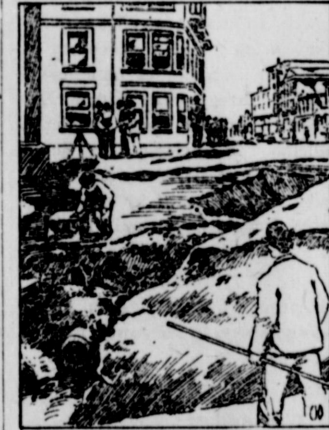
SAN FRANCISCO FLATS SUNK ONE STORY INTO GROUND.
