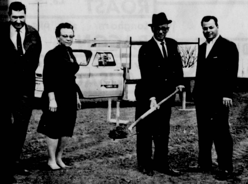
GROUND BREAKING CEREMONY--Mayor S. W. Ross turns the first construction begins on Mar- rusing Home. The $157,000 home off the southwest corner of High School, west of the location
