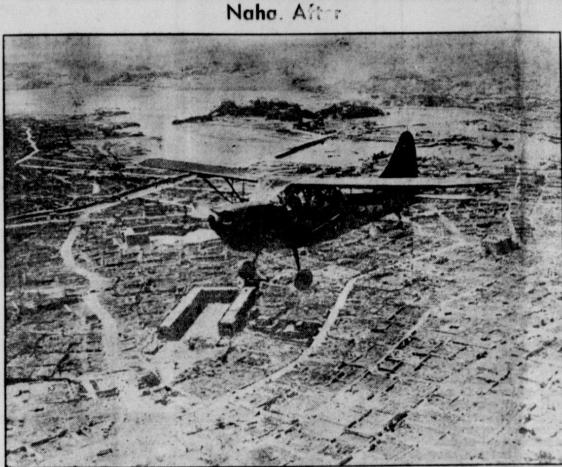
Only a few of the stouter buildings still stand in Naha, Okinawa capital where 65,000 people lived, after the terrific warfare waged there by the 6th Marines. Sunk ships show in the harbor beyond. The plane is a Marine observation craft. (Marine Corps photo.)
