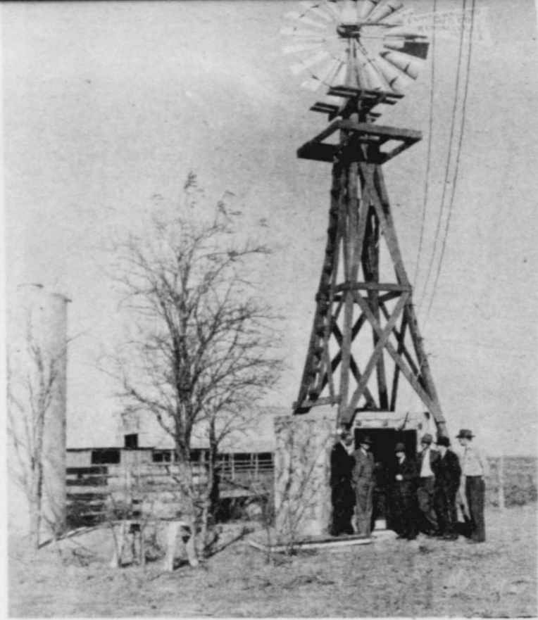
This picture was taken in 1940 at the A.H. Kreis farm eleven miles east of Floydada. On this occasion one of the first deep well installations was converted to electricity. This pump is set at 225 feet and powered by 1 1/2 HP electric motor. In the picture from left to right are: A.H. Kreis; Edgar Kemp, Soil Conservation Service; Clifford Tubbs, County Judge; Henry Schact, Board member; L.A. Williams, AAA county committeeman; and L.W. Chapman, Co-op manager. Mr. Kreis was a Board member at this time too.
