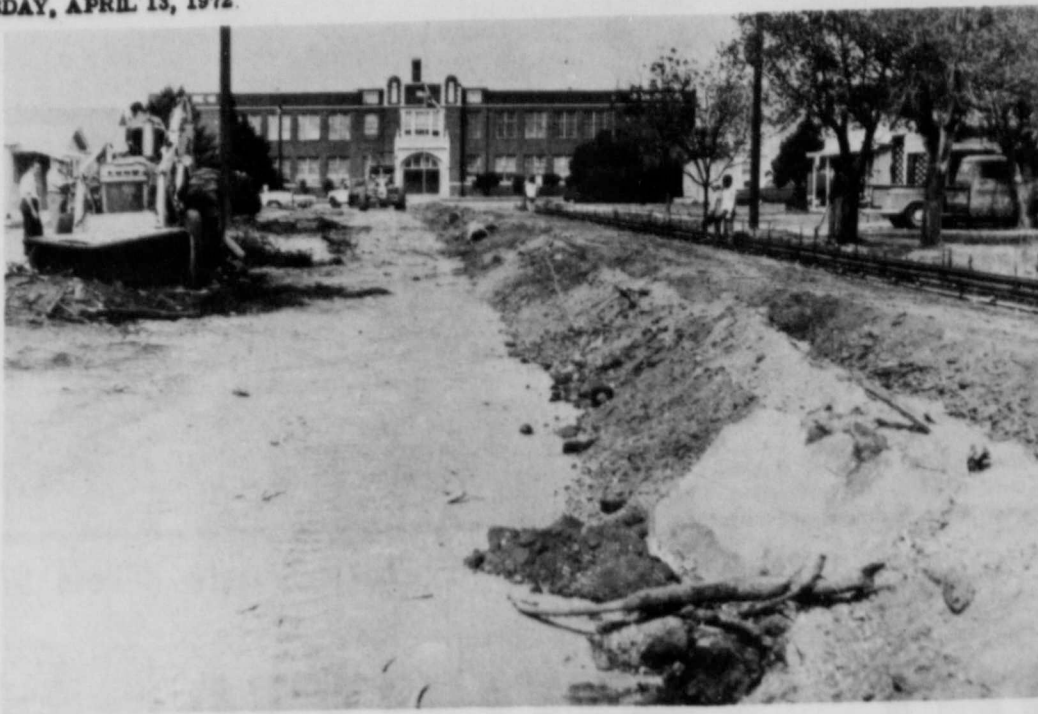
CITY STREET PAVING BEGINS . . . Workmen began preparations for complete paving and curbing of three blocks of Floydada streets this week, on Jeffie Street a block east and a block west of Junior High School and Hallie Street between Main and Wall. Along with the complete paving of those three blocks, seal coating is planned for some 43 blocks of Floydada streets, and the Floydada Municipal Airport ramp and runway. The paving operations will probably be completed by May 15, weather permitting, according to city manager Bill Feuerbacher. (Staff Photo)
