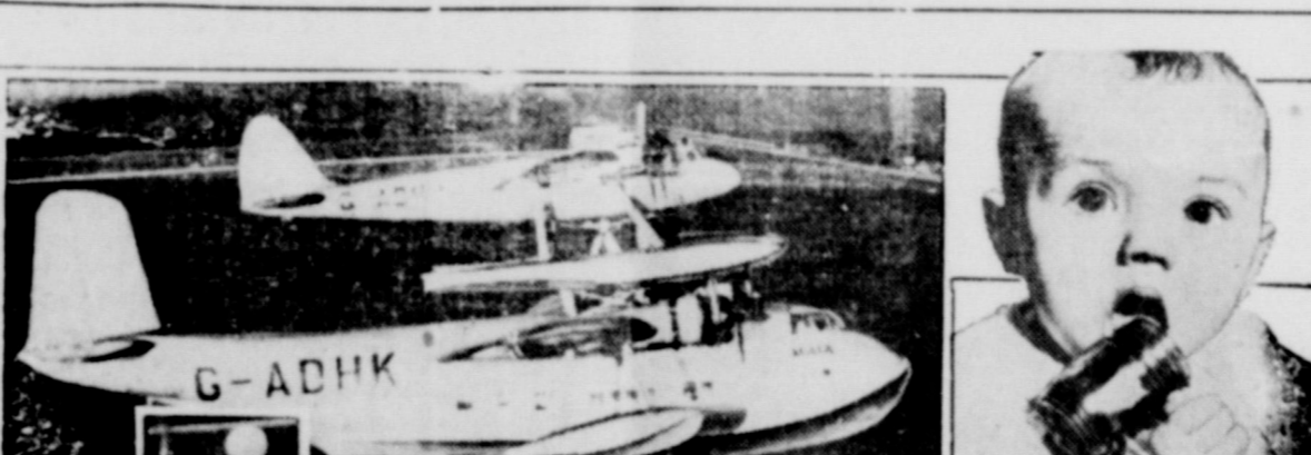
AERIAL HITCH-HIKE... Revolutionary 'pickaback' airplane, shown here in test at Rochester, England, takes off as one plane, lands as two, for small seaplane can leave 'mother-ship' at 700 feet.
