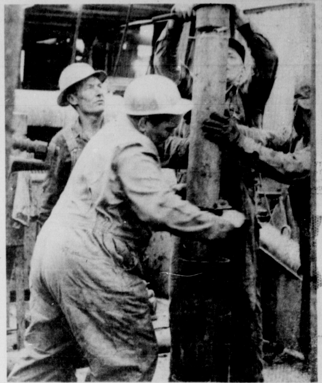
A FINAL CHECK . . . The day crew on the London wildcat make up a test tool in preparation for a drillstem test. The crew started in the hole with the tool Tuesday evening. Results of the test will determine if any further work is warranted on the hole.
