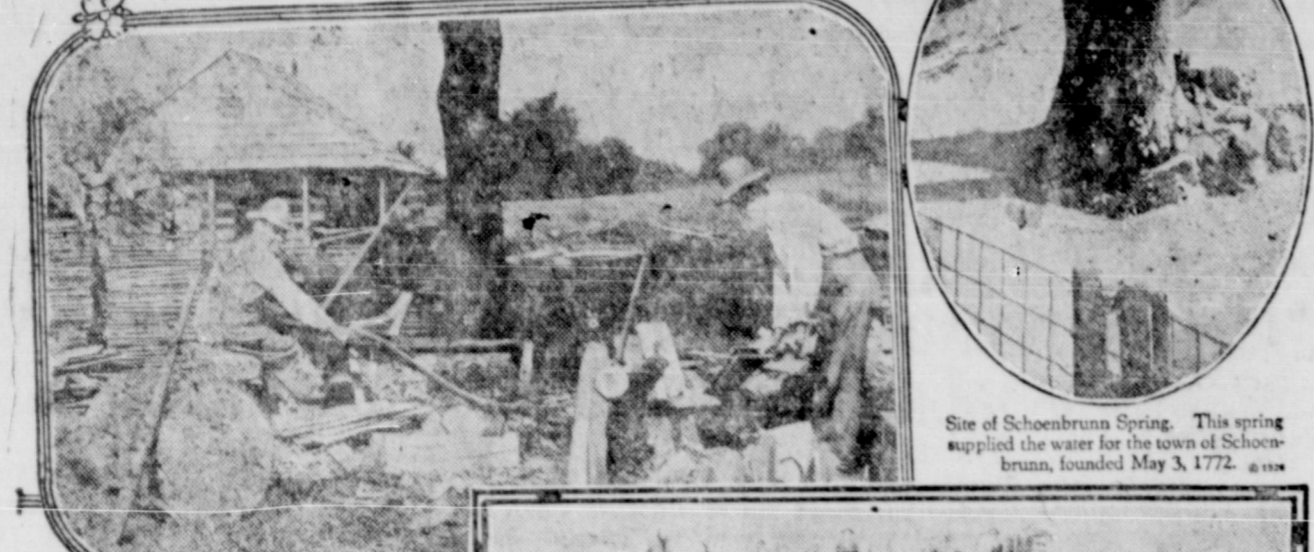
Splitting and shaving shingles—pioneer style—for school house, Sept.-Oct., 1927. Schoenbrunn Memorial Park, near New Philadelphia, Ohio.
