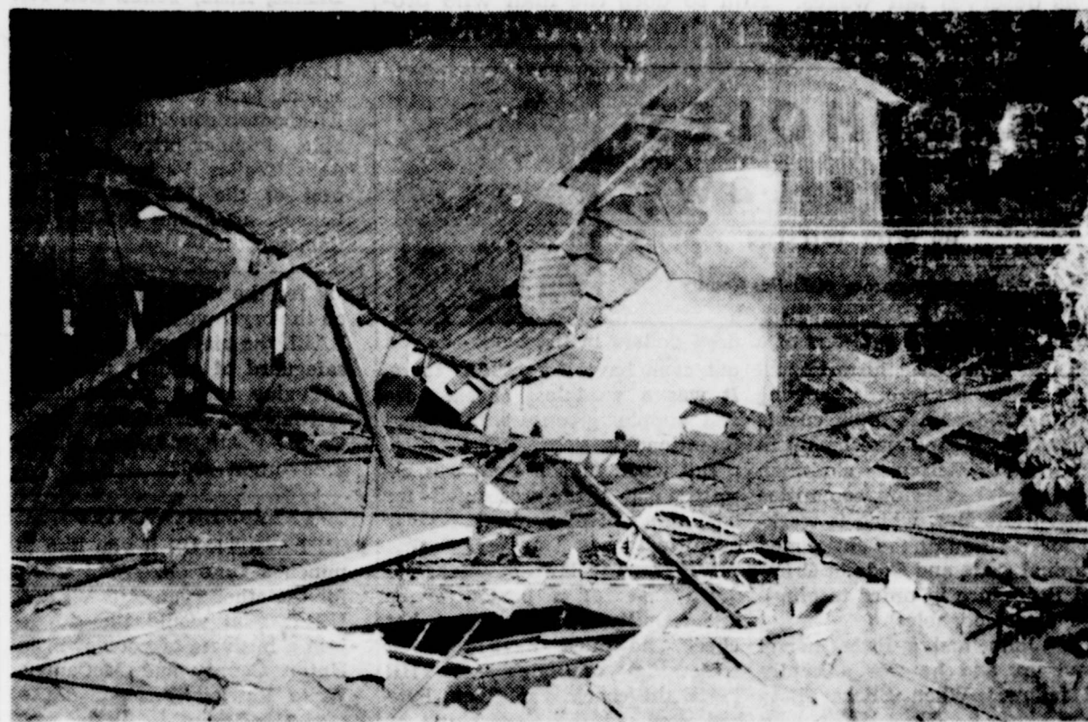
The home of Mr. and Mrs. J. W. C. Hayes was virtually demolished by gas explosion last Tuesday night. Shown above, the fire in the front portion of the building is still burning, while the partition at the rear of the house still standing was torn apart. Three members of the family who were in the building at the time of the explosion escaped without serious injury. The home was located behind the West Texas Utilities office in downtown McCamey.—Photo by Johnson.
