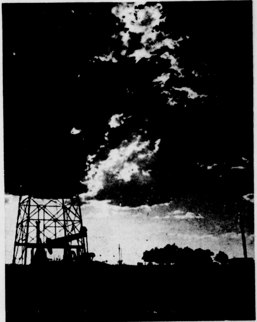
A DISAPPEARING SCENE —Derricks such as these are in the twilight of a fabulous career. In the past derricks were left at well locations for use if it was necessary to work over the well in the future. Now a portable workover rig is in general use. This derrick, near Big Spring, Texas, will probably be torn down as will many others like it as the industry moves ahead into another year of progress.
