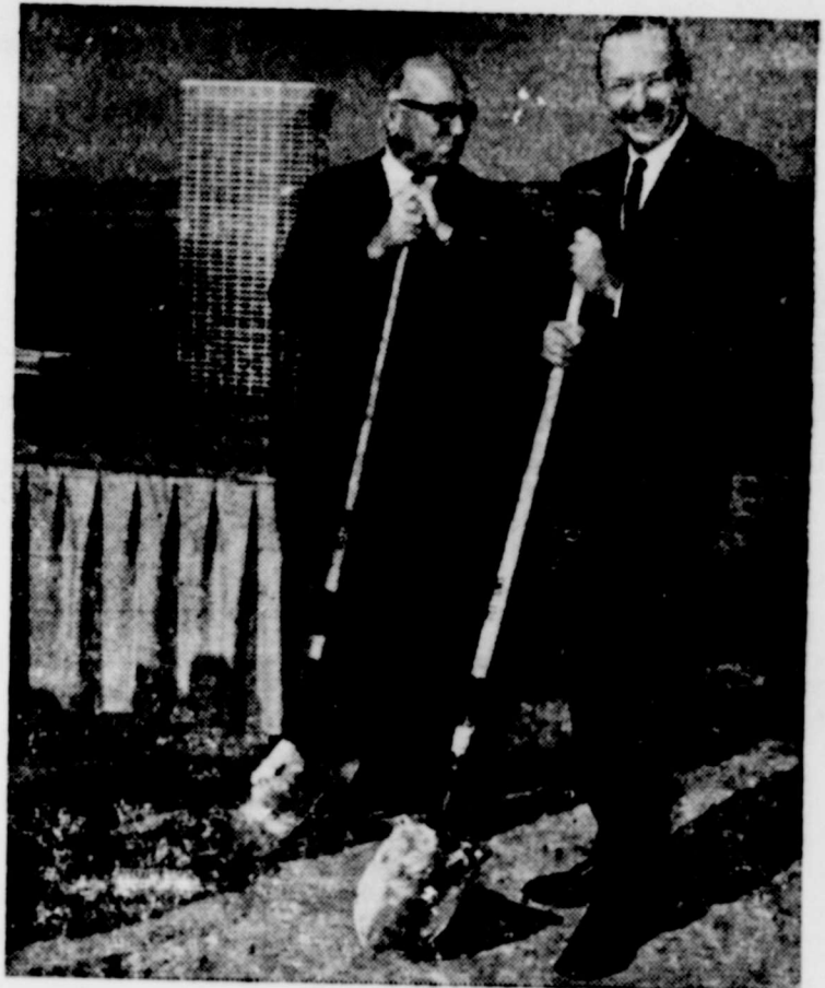
SPADEWORK ON HUMBLE'S NEW HOME - In Houston Morgan J. Davis (right), president of Humble Oil & Refining Company, turns the first shovel of soil for Humble's new 44-story office building shown in the background model, while Humble Division President Ray H. Horton joins in the ceremony. The 600-foot structure, with some 1,000,000 square feet of usable space, is scheduled for completion in late 1962.
