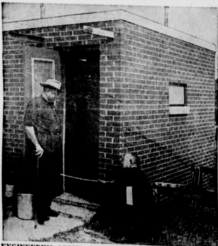
ENGINEERING ADVICE on how to add an entrance baffle to his new fallout shelter is obtained by Carl L. Underhill (left), of Raleigh, N. C., from Archie W. Green, Jr., engineer for the North Carolina Civil Defense Agency. Underhill discovered that a baffle was needed to block dangerous levels of radiation which, after nuclear attack, could penetrate a normal door of this $1,600 shelter. Green was hired early in 1961 under a Federal program to pay half the costs of new civil defense employees. (OCDM Photo)
