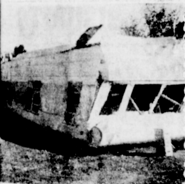
HOUSES found the going particularly hard Friday as three were completely overturned—the most severely damaged. Several others were moved about and practically all in town had hail damage.
