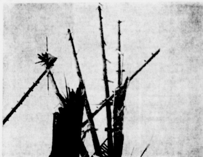
FIFTEEN-INCH-THICK poles were snapped like match sticks at the Hilltop Drive Inn where their opening had been only a matter of days away. Re-construction work was started immediately on the scene.
