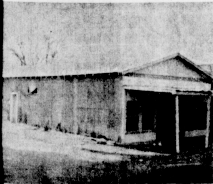
Work was completed last week on "lifting" the upper half of the two-story Odd Fellow and Rebekah Lodge Hall, reducing it to the structure shown above. Funds from the football concession stand operation were earmarked two years ago for the work and further improvements to the front and sides are planned.
