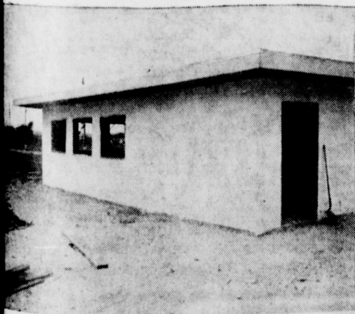
... Work almost finished
