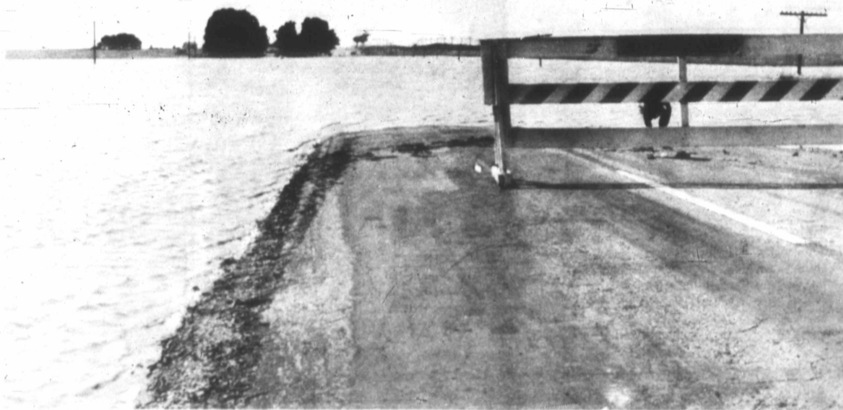
MAN THE PUMPS — This highly publicized section of U.S. Hwy. 84 became a fair-sized lake last weekend and halted traffic on the highway for an indefinite period. Rains last Thursday, Friday and Saturday in the area totaled from three to eight inches, with the biggest single rainfall Friday. Most cotton in the region was washed out, and farmers already were replanting this week as soon as they could get in the fields. Some fields and this part of the highway remained under water. Traffic was being routed around the quarter-mile-wide lake. (Staff Photo)
