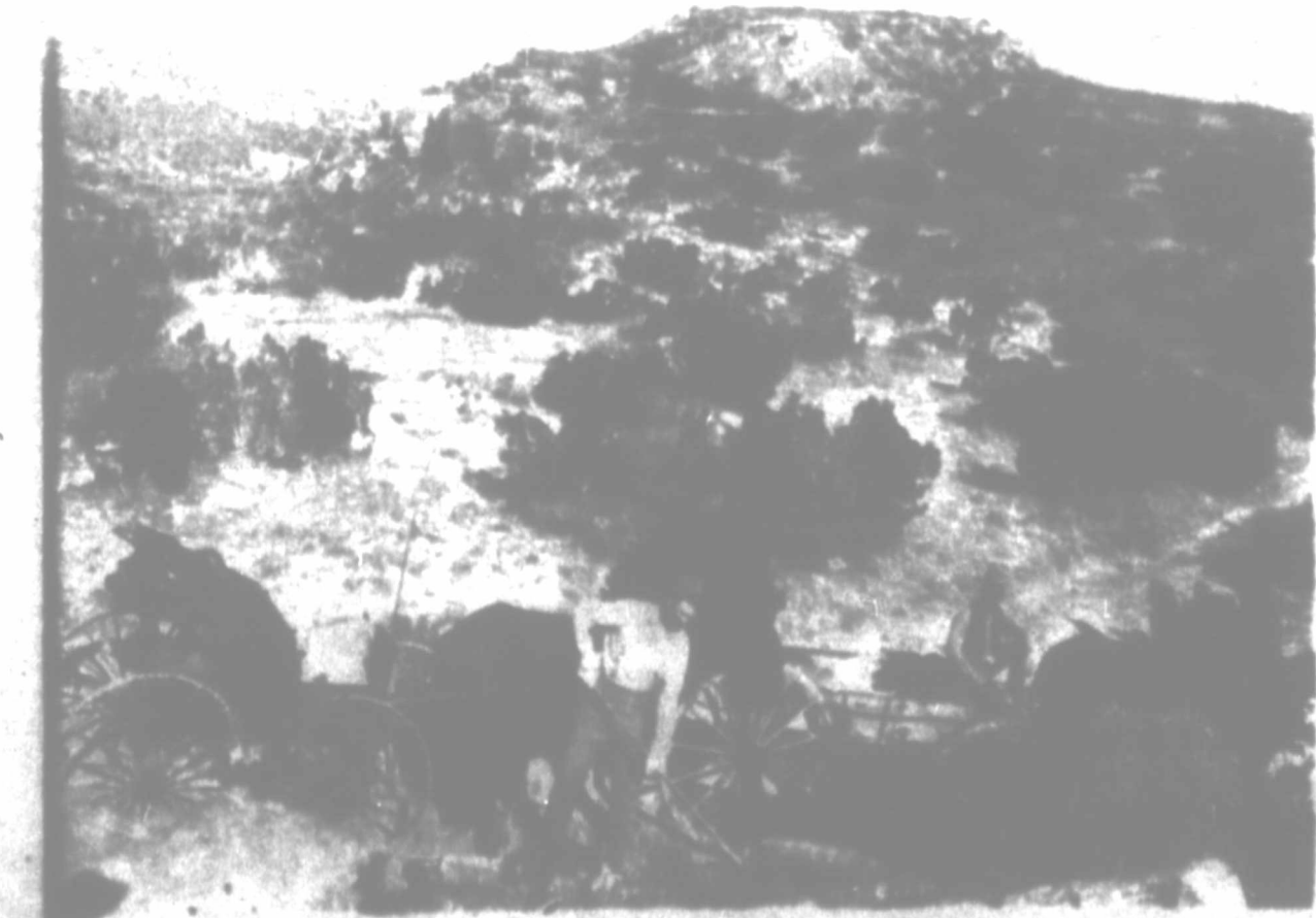
ROAD BUILDERS -- This early-day photo taken around 1912 shows workmen clearing boulders from the path of Schott Road when it was under
