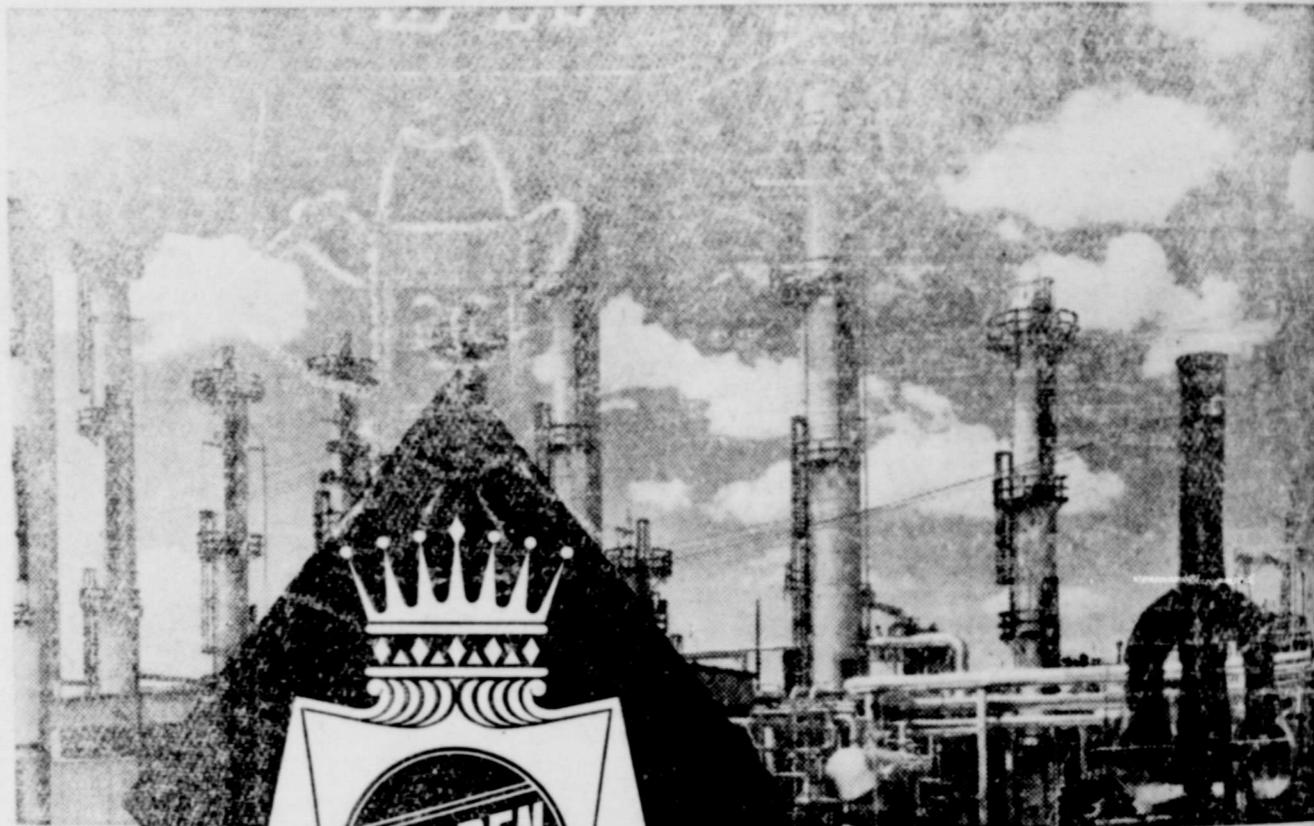
PARTIAL VIEW OF COSDEN'S MULTI-MILLION DOLLAR REFORMING UNIT
