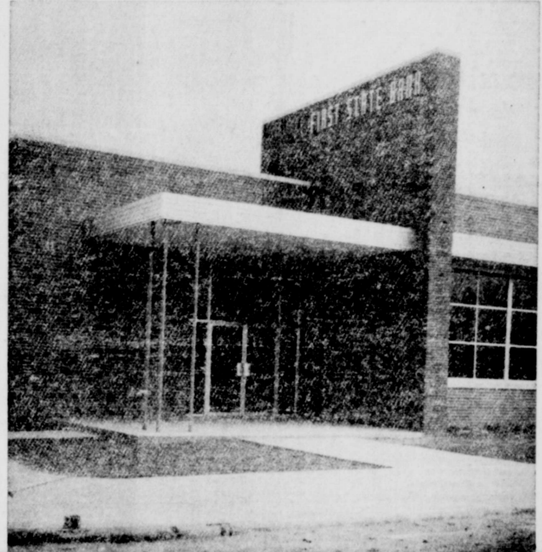
TO OPEN HERE SATURDAY — One of a series of photos taken by Norman Studios shows the ultra modern designing in the structural layout of the new First State Bank which is to have its grand opening here Saturday afternoon.
