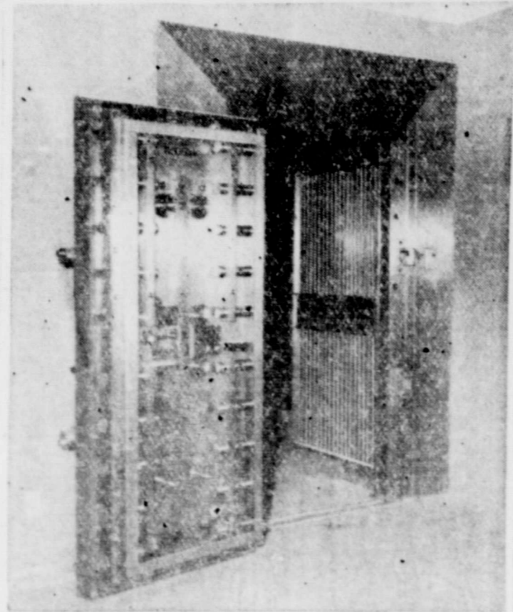
SAFETY FIRST — the giant door that guards the vault in the all new First State Bank, Morton. By Diebold of Canton, Ohio, the vault door, with safety deposit boxes just beyond, will be just one of the many modern banking methods to be viewed Saturday.
