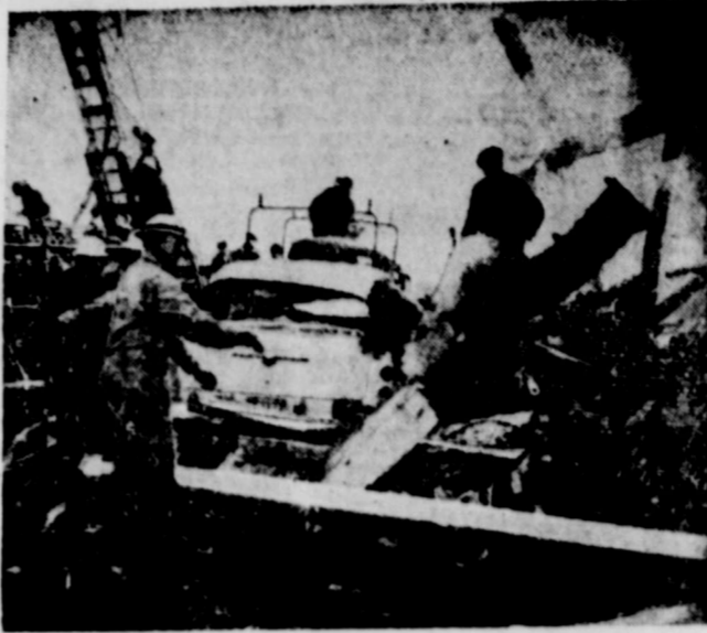
BLAST DEBRIS is cleared away in Reno, Nev., by members of Ecco Rescue Unit No. 1 of Washoe County Civil Defense after a gas explosion which rocked downtown Reno last February 5 killing two and injuring 68. The CD workers, trained to meet similar situations in time of war disaster, found the body of one of the victims under the car flattened by blast. (Photo by Gene Christensen, Reno, Nev.)
